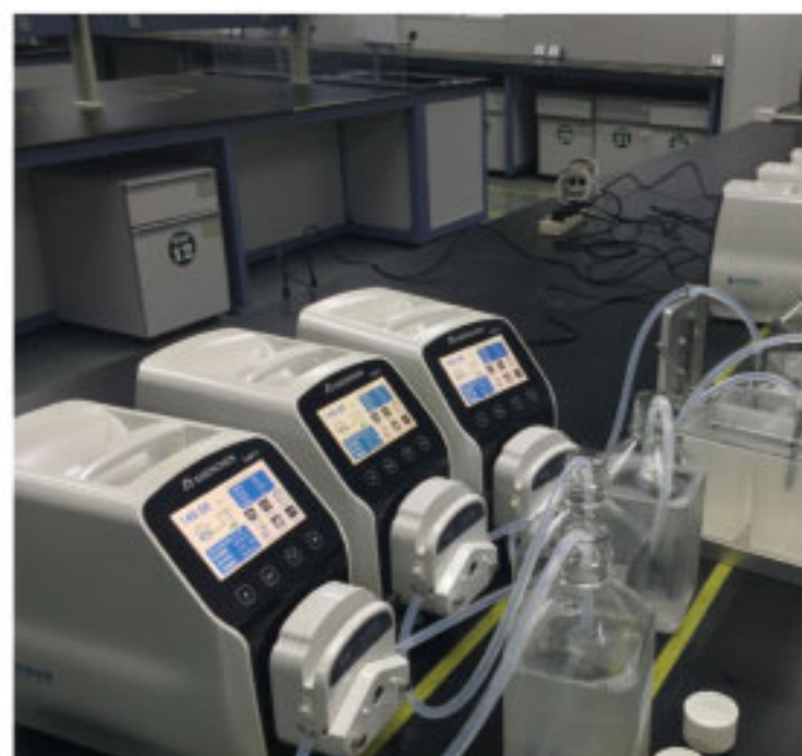
Laboratory chemical dosing
